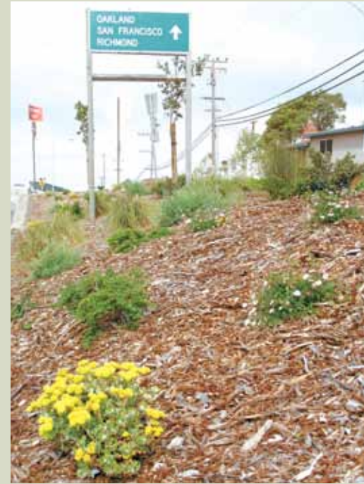
Left: Albany Buchanan Street medians were constructed using sheet mulch and other Bay-Friendly landscaping practices.
