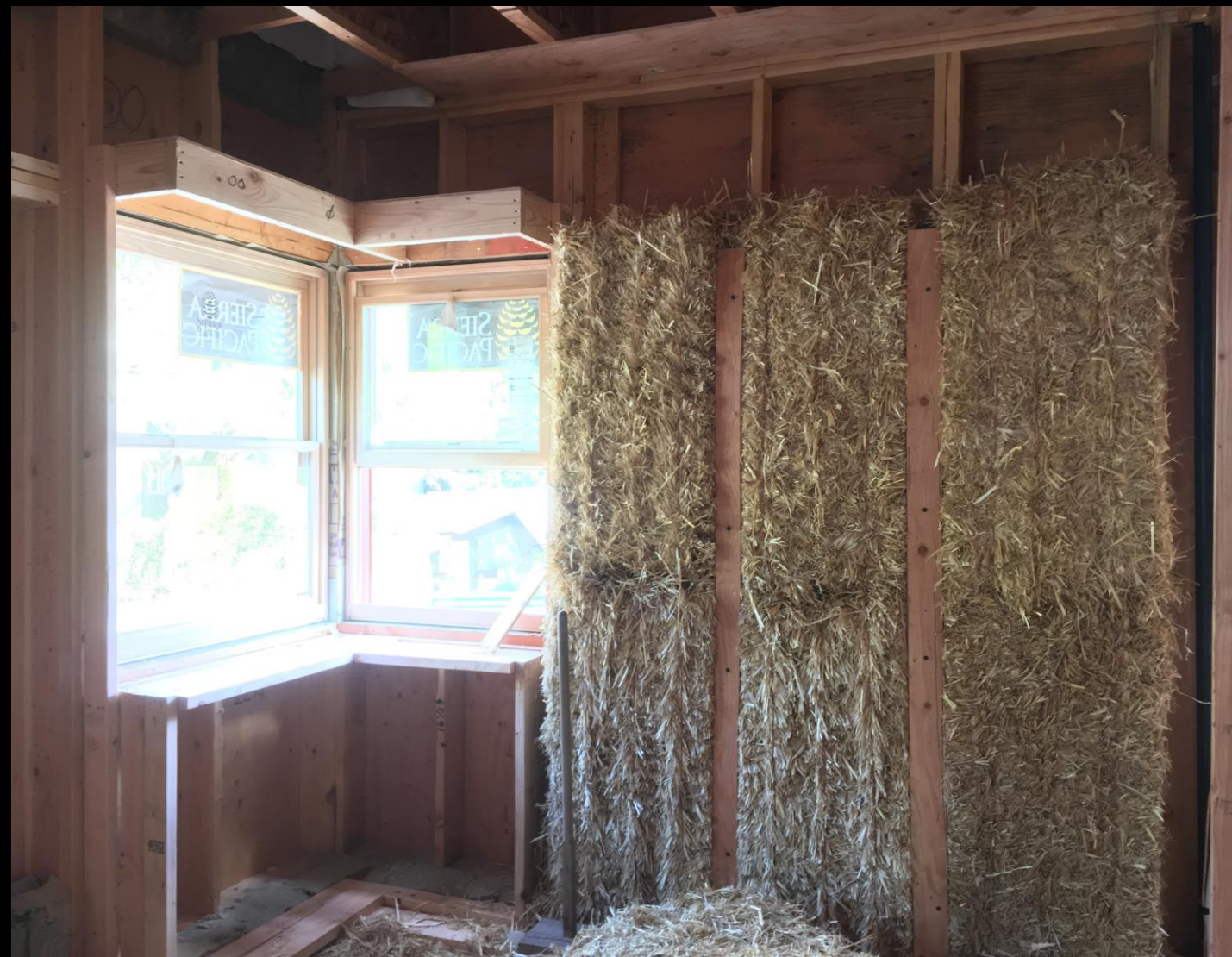
BOEBS – Bales On End Between Studs
